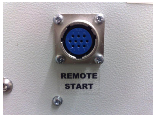
Remote start connection point – located on front of unit
